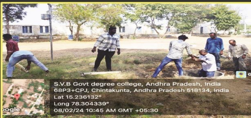
Staff and students participated in construction of water harvesting pit on 08-02-2024
